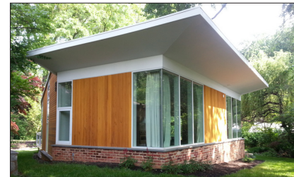
3306 Pendleton Drive (1950), Top: street view; Bottom: rear addition. Michael Cook, architect. Photos: Michael Cook
